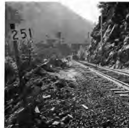
MILEPOST 251: Looking west toward the East portal of Tunnel 15. The intermediate signal (rear center) is located on an 8°45" curve. Note the slide fence at the right. The Buck's Creek power station is located off to the left.
