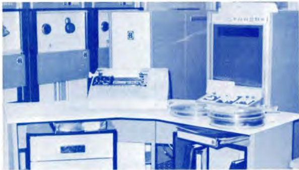
The Burroughs-3500 "master control" is the brain of the system. The electronic typewriter gives commands to the entire system.
