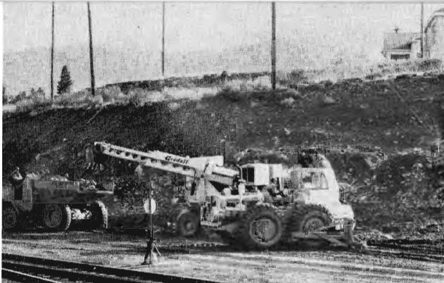
John Aughe, George Blackwell, and Hoyt Stewart operate a Gradall, Tournadozer and Dumpster to construct a ditch between the depot and shops at Portola. The ditch will carry away casual water which forms in the parking lot and road. Jack Miller photo.
