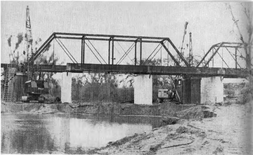
Looking downstream showing temporary dam, later opened so flow of water will be diverted from wooden trestle to pass between new concrete piers.
