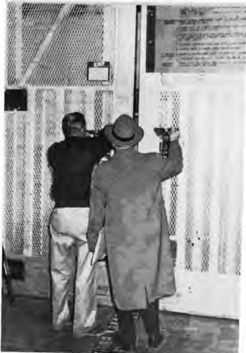
After opening these WP compartmentizer car gates, inspection revealed no damage or shifting in load.
