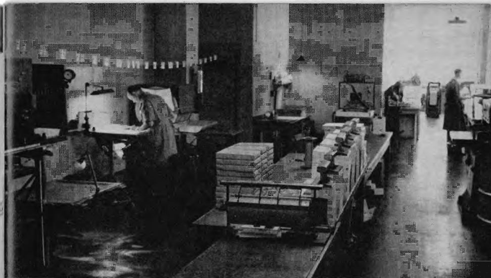
Over-all view shows photostat camera, retouching table, pako dryer at left; padded forms under rail weights, center; cutter, Xerox machine and offset presses at back on right.
