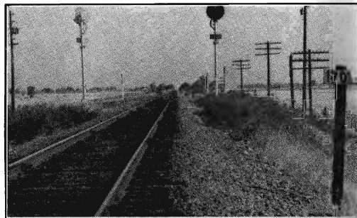
*Milepost No. 170: Looking east toward East Arboga, two and one-half miles beyond.
