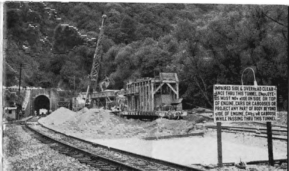
Looking west into tunnel, in foreground is cement slab poured from waste concrete used for storage of aggregates, "Pumpcrete" machine, mixer, "Bin-an-Batch" and crane.
