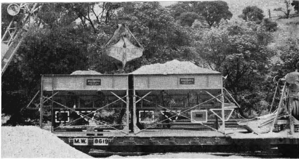
Loading aggregates into "Bin-an-Batch." White dotted lines indicate path of measuring device, shown by solid white lines at right of machine. Accurately mixed aggregates are weighed before dumping into bucket at right which carries them to mixer at extreme right.
