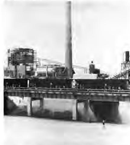
*As the coal unit train moves across the trestle its cars are automatically unloaded through dump bottom doors. Nozzles under the trestle spray the coal with water to prevent dust. The train will make three deliveries a week at the North Valmy Generating Station in Nevada. (Union Pacific Railroad photo)*
