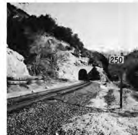
**MILEPOST 250:** A view of the east portal of Tunnel 15. Tunnel 15 is 3117.8 feet long and was constructed in 1956 after the massive flood of 1955.
