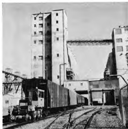
Grain cars are unloaded at a rate of about one every five minutes at the port's grain terminal. It will take about two days to load the grain ship to its capacity.
