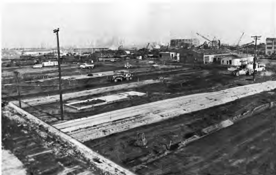
The distribution site under construction in this early January photo is where the roundhouse and repair shops were formerly located. Photo: Andy Parsons.
