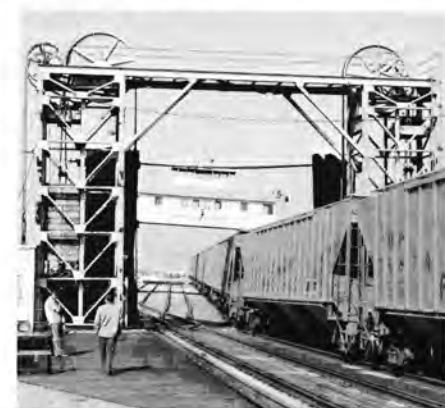
Grain covered hoppers on arrival at Oakland are loaded onto WP's ferry, MV Las Plumas.
