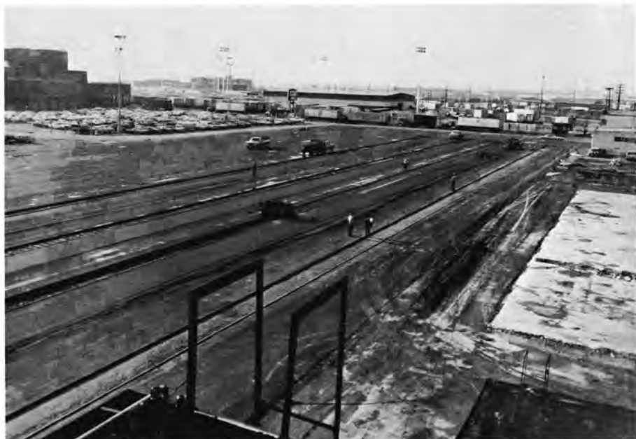
Final paving for the new unloading area transforms the old maintenance tracks for the California Zephyr into the new distribution site.
