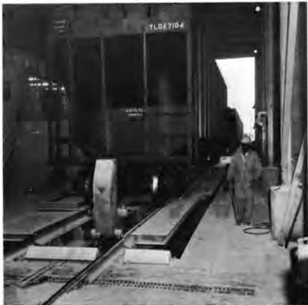
A covered hopper car is weighed at the San Francisco grain terminal before unloading.
