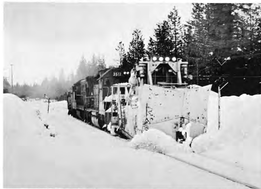
Backed by two 3,000 HP, WP locomotives, maintenance of way spreader #7 plows the snow along the main line of the inside gateway near Greenville. Photo: Dale Sanders.
