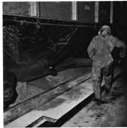
Workmen open the doors under the covered hoppers to unload the corn at San Francisco. Corn flows by gravity to the belts below which take it to the tops of the storage elevators.
