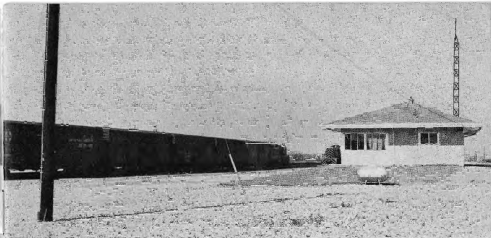
Freight cars leaving the Ford plant pass WP's new Milpitas office. The 30-foot self-supporting radio tower affords rapid communication between office, crews, the Ford plant, Niles and San Jose.
