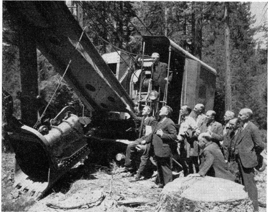
GROUND BREAKING — The cut above shows the first power shovel on the Bieber Line digging in at M. P. 17.5 near Greenville, August 16, 1930. The late Harry M. Adams, then president, is at the controls. Below (left to right): Thomas P. Brown, publicity manager; the late Harold K. Faye, freight traffic manager; R. A. Hollenbeck, division engineer, Elko, then construction engineer, Westwood; Thomas L. Phillips, now chief engineer, then principal assistant engineer in active charge of the project; the late Col. J. W. Williams, then chief engineer; H. V. Johnston, resident engineer, Greenville; Charles Elsey, now president, then executive vice-president. In the foreground: the late Bode K. Smith, passenger traffic manager (seated), and D. C. De Graff, general auditor.
