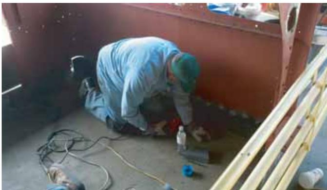
Dick Coudin drills holes for rivets at the base of the cab.
