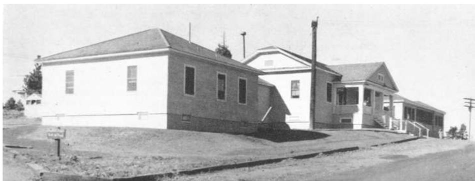
This 1957 view of the hospital shows the newly installed siding and what appears to be a new roof. Exterior and nterior surfaces had also just been repainted.
