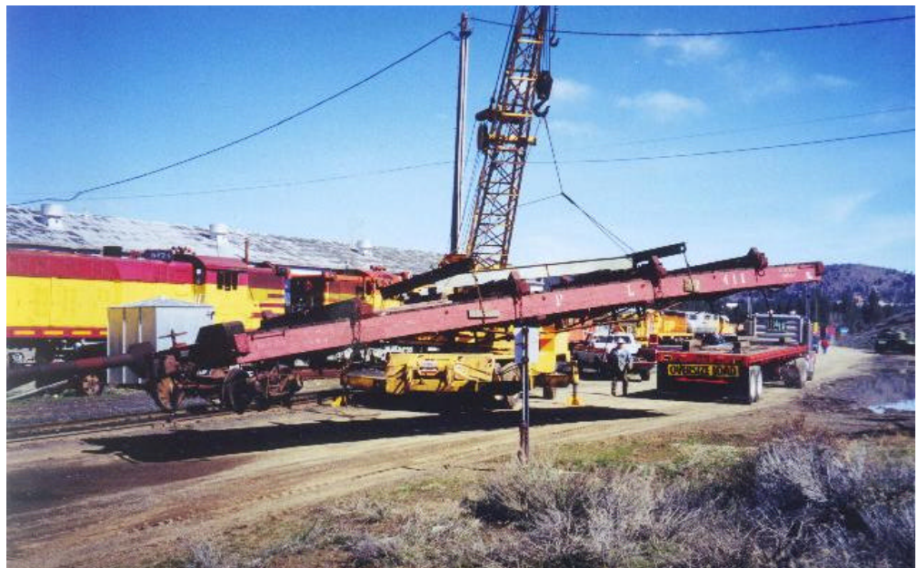
After being lifted from the truck trailer one of the flat cars is being swung around in preparation for setting it back on its arch-bar trucks. - Norm Holmes
