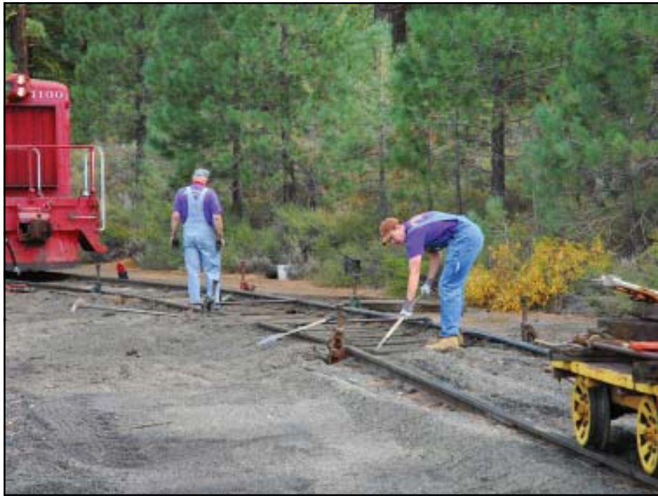
Track laying and maintenance continues to this day. Here volunteers fix a low spot on the balloon.
