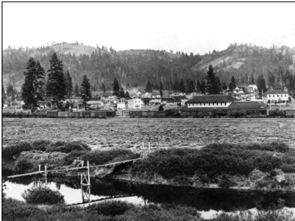
Similar view. Footbridge over Feather River in foreground.
