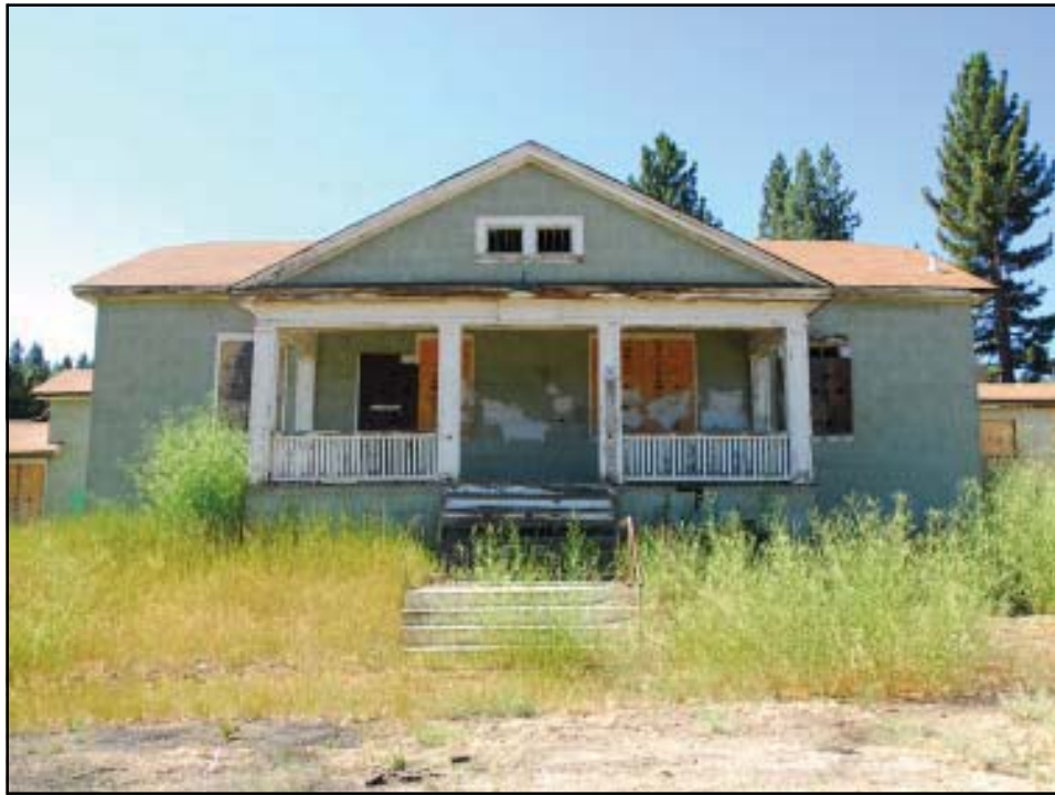
Original 1912 hospital building on August 6 th of this year, just before the annual summer's-end brush clearing by the California Conservation Corp.
