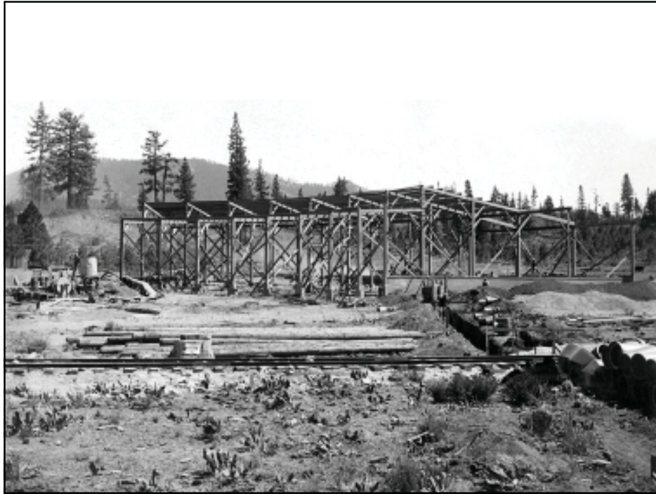
Roundhouse construction August 1909
