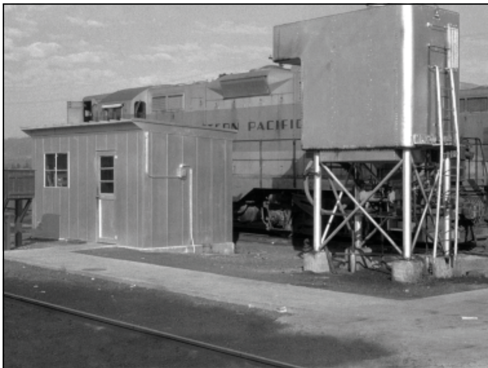
Waste oil tank made from the oil bunker from a retired steam locomotive tender.
