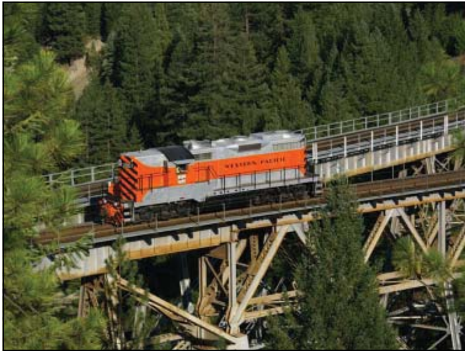
2001 returning to Portola light on the Spanish Creek bridge near Keddie.
