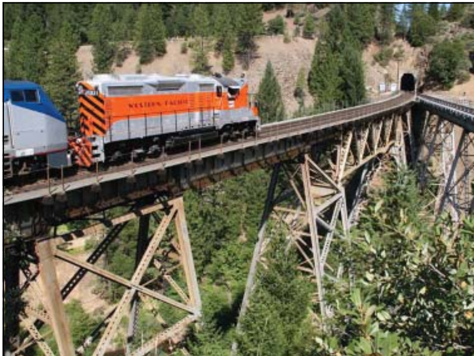
FRE at Spanish Creek Trestle near Keddie.
