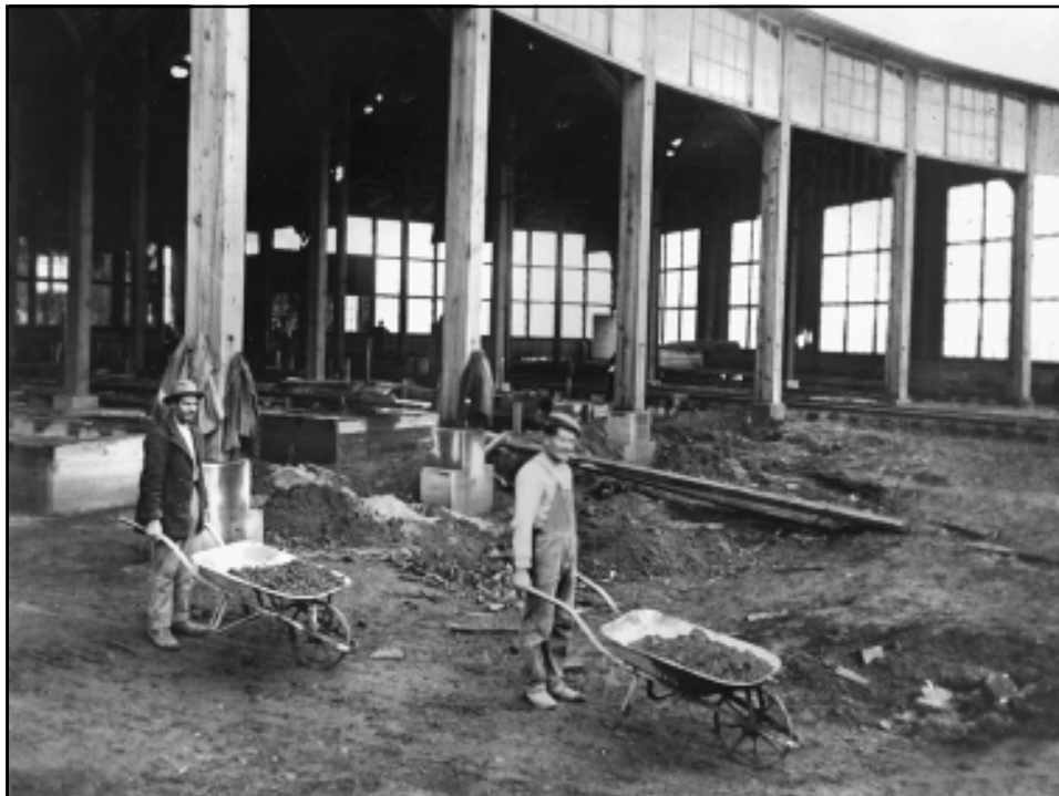
Roundhouse construction August 1909. Roundhouse had concrete pits with a dirt floor.
