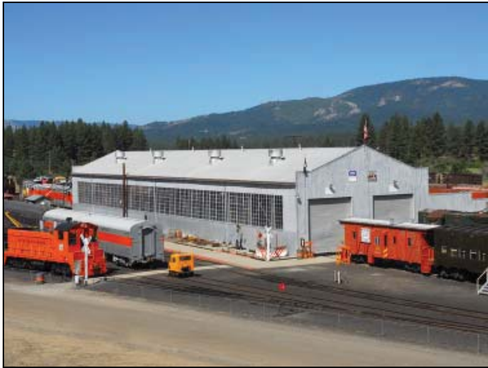
The 225-foot, 16,000 square foot diesel shop is still the centerpiece of the facility.
