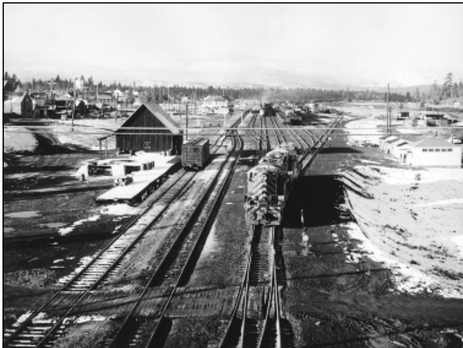
Looking west from the Gulling Street overpass. Yard on right. Freight house on left. House track off main just west of freight house. Depot in background to left of main,
