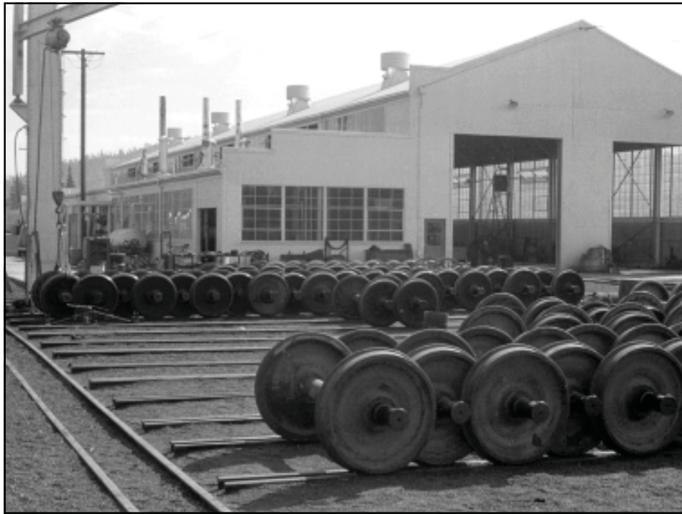
1955 view of west end of diesel shop, wheel hoist and spare wheel sets.
