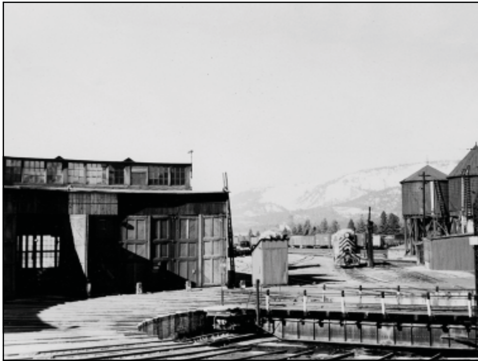
WP Geep sits in a steam-era facility shortly before the roundhouse was dismantled.
