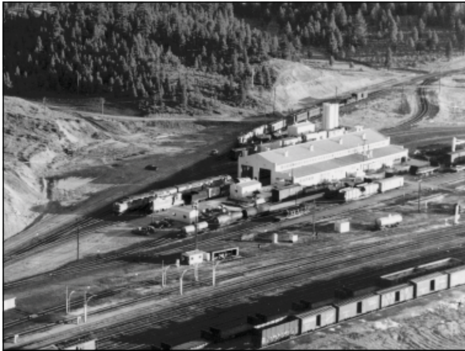
Close up of diesel shop.
