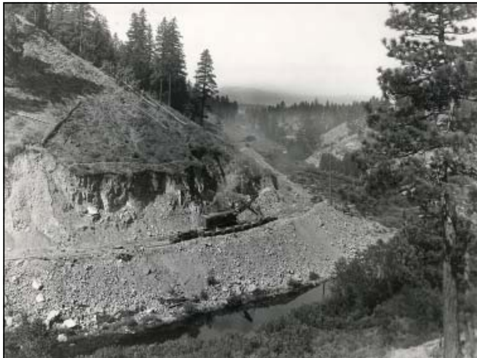
Rebuilding B&L ROW at Rocky Point.
