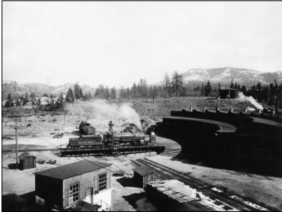
WP 319 takes a spin on the 110-foot turntable in front of the expanded 12-s tall roundhouse. View likely taken from the top of the fuel-oil tank.
