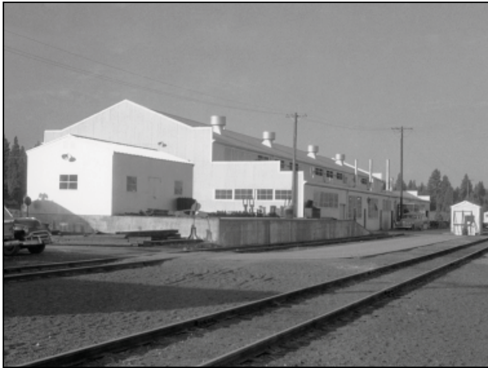
1955 view of east end of diesel shop and loading dock.
