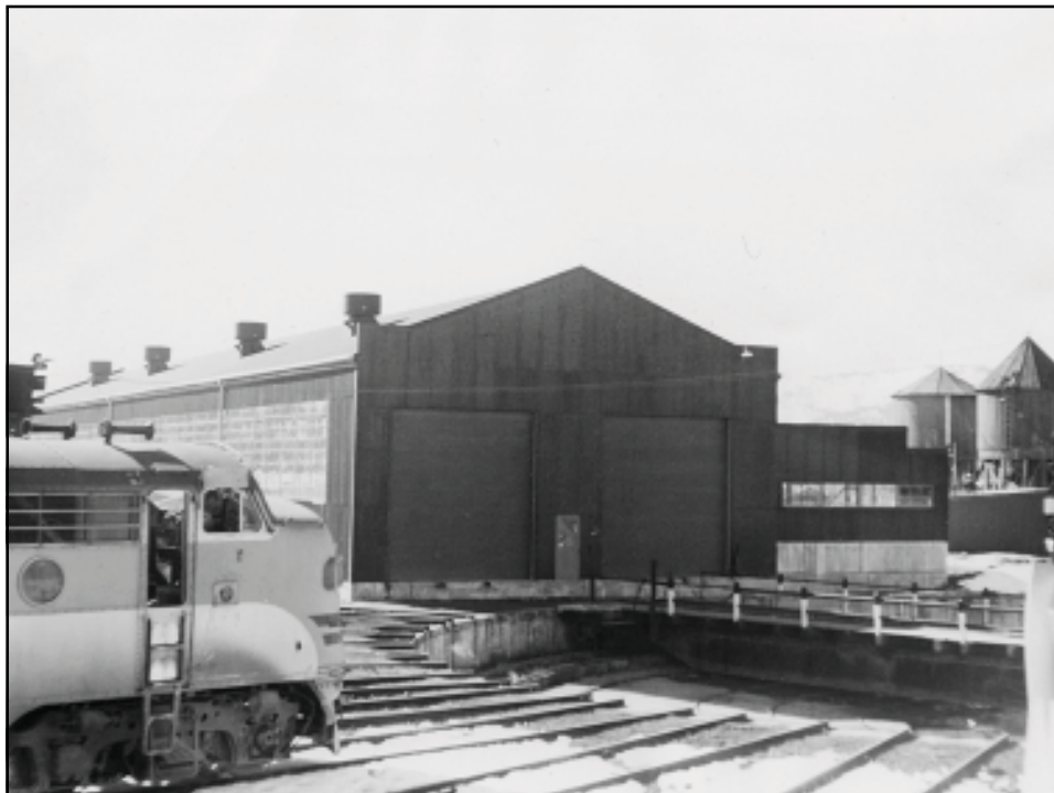
New diesel shop during construction with turntable and whisker tracks still in place.
