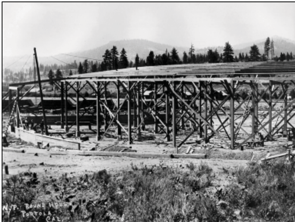
Roundhouse construction August 1909
