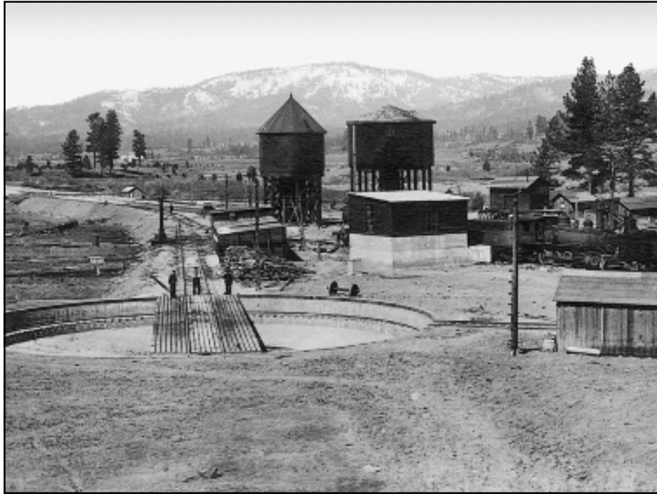
Early view of turntable, original water tank, fuel-oil tank, oil house, and sand bin. WP 124, former B&L 2-8-0 oil burner.
