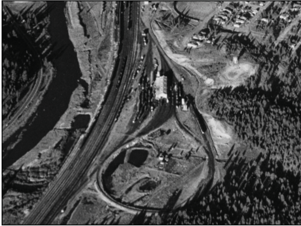
Close up of balloon track and diesel shop.
