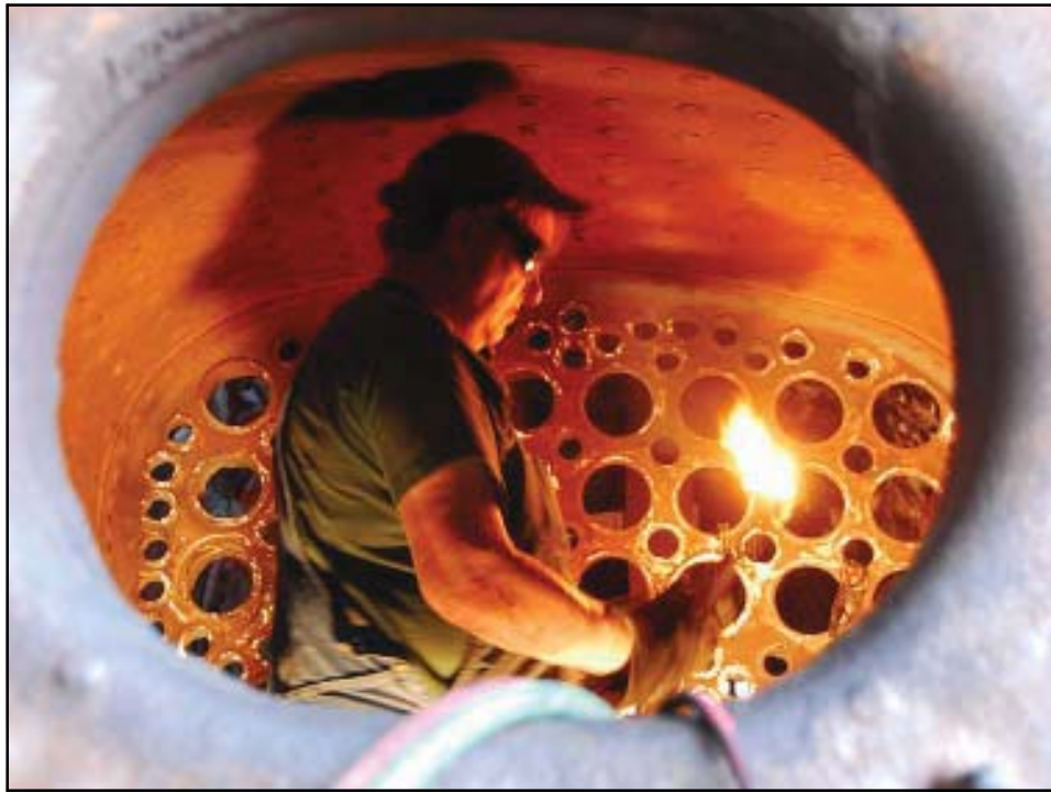
People can be found in every corner of the facility working on something. Here is work being performed on the tube sheet in the 165.
