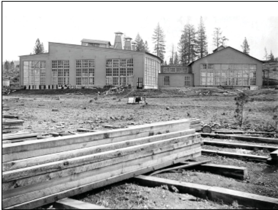
North side of roundhouse later during construction. Boiler room and machine shop attached to rear of roundhouse.
