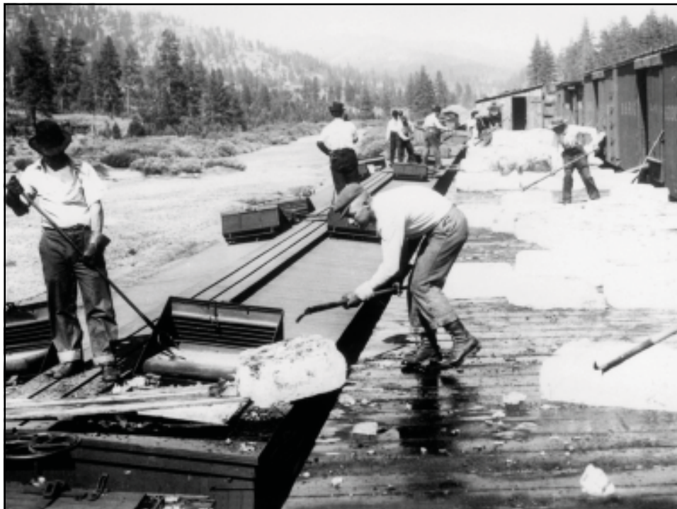
Reefer icing platform in east Portola circa 1915. Cars of ice came off the B&L from Gulling and were unloaded on the high track on right. Reefers spotted on ice deck rail next to main.
