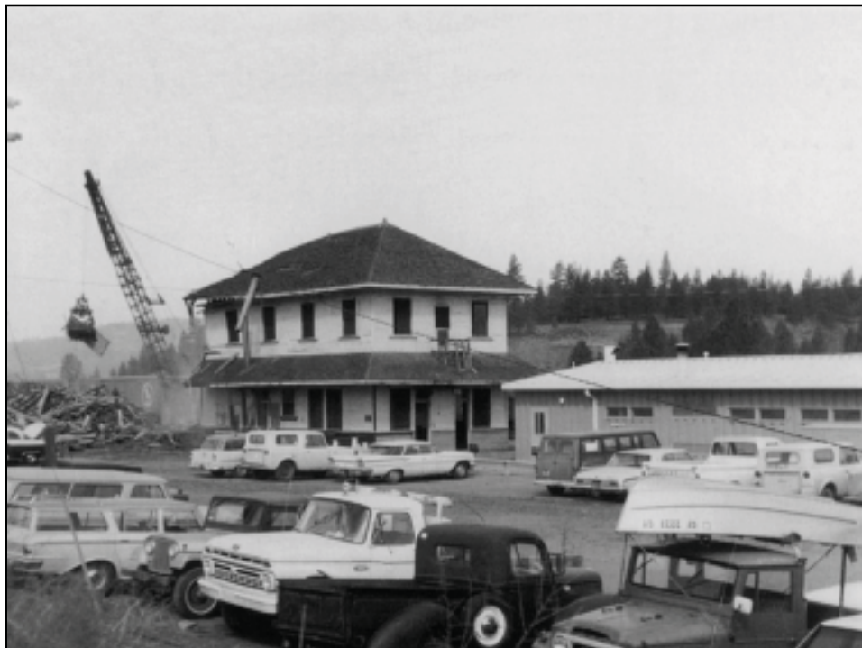
Old depot coming down with new depot just east of it.
