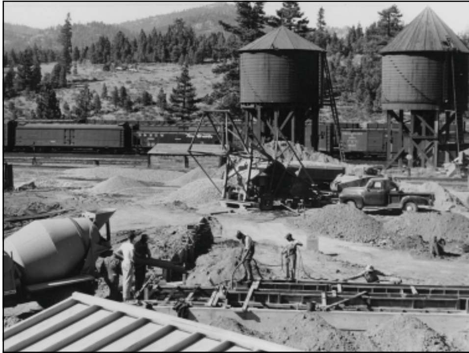
Pouring the cement foundation for the new diesel house. Machine in background is called a Jiffy Batcher for mixing concrete.
