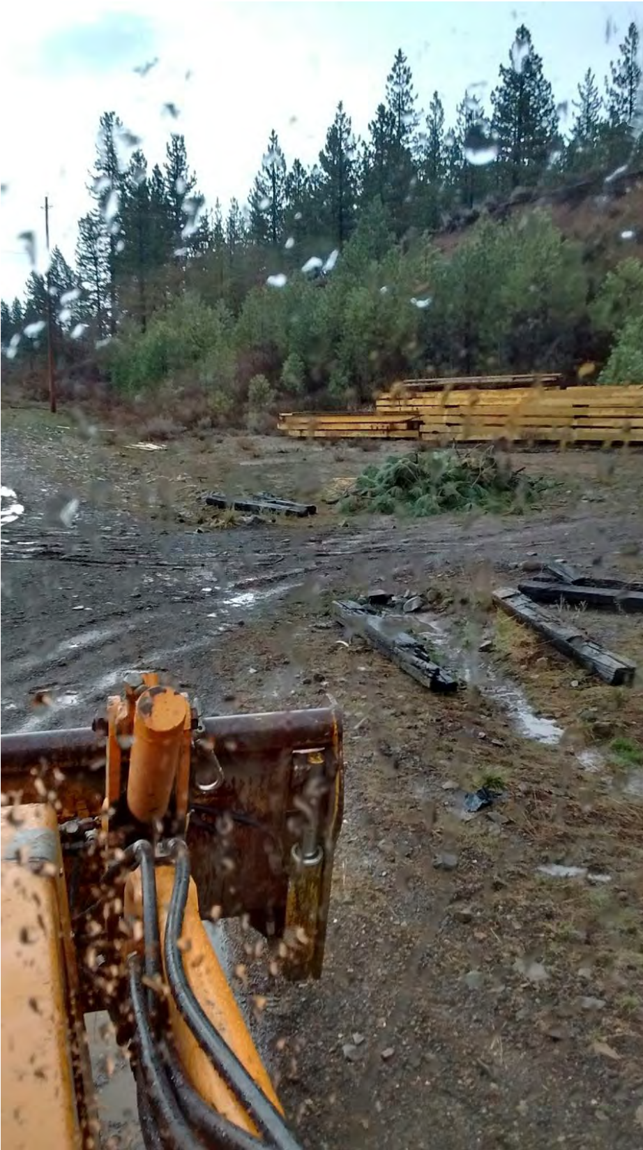
Not the best shot, but shows the ditch along foamer ally. Had to remove debris from around inlet and outlet of culvert under road. Runs well enough to drain out now rather than be a long narrow puddle.
