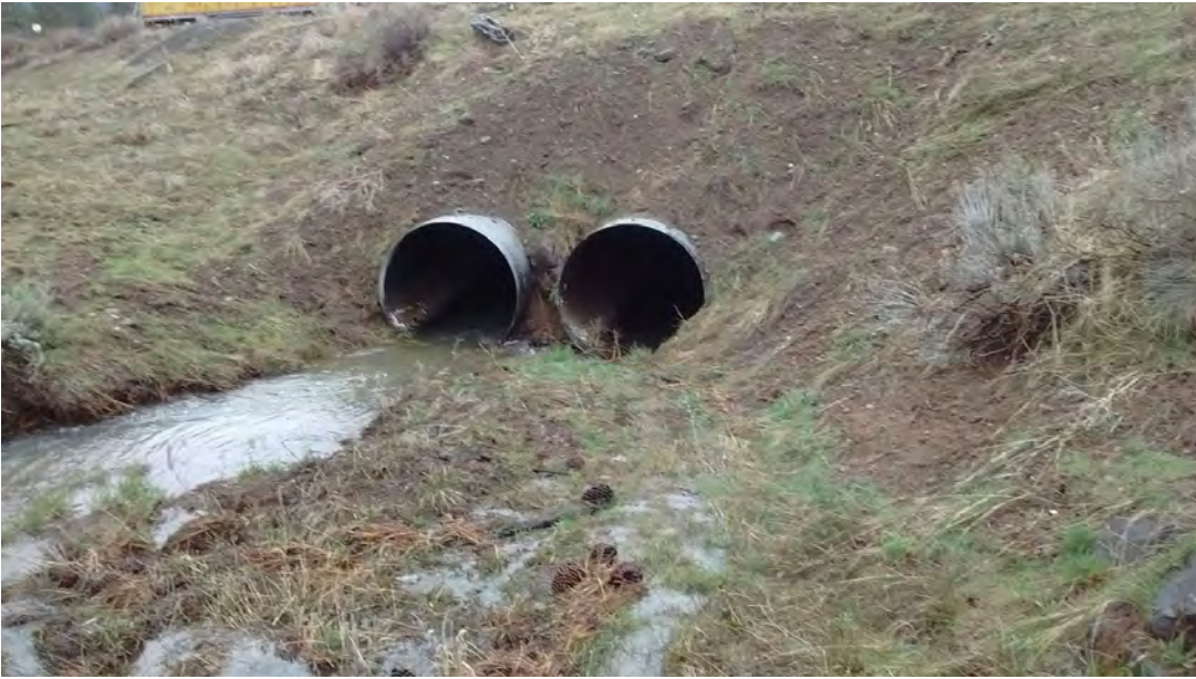
Previous photo and this one show the culvert on the north side of the balloon near the 2/3 switch. East culvert here is in the early stage of being undermined by creek.
