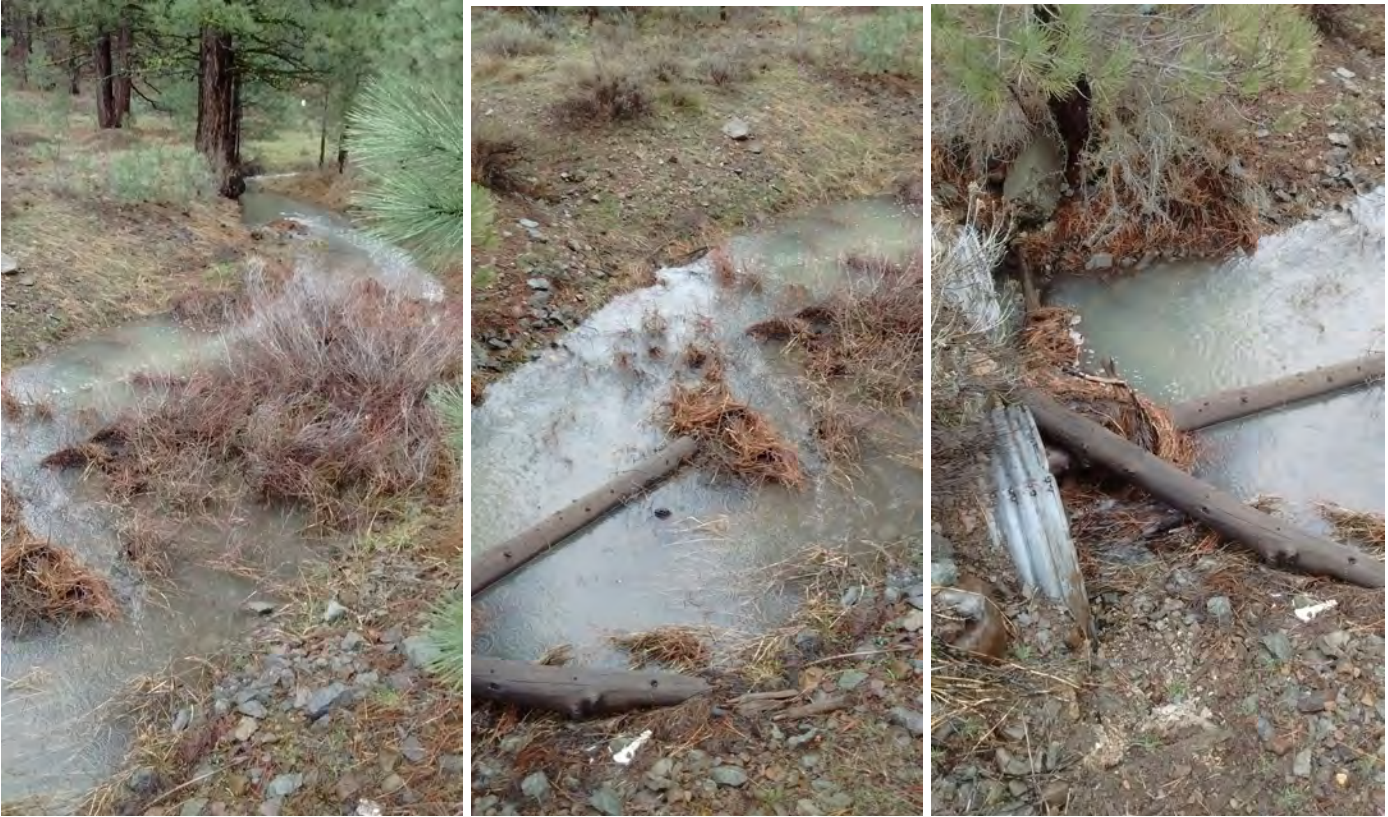
South Side Milward Culvert before Mitigation
