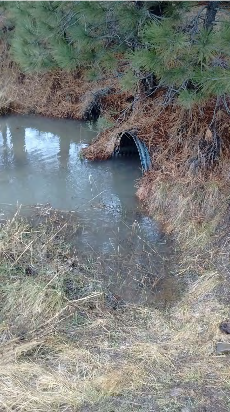
North Side of Milward Culvert. Tubes are clear and running fine.
