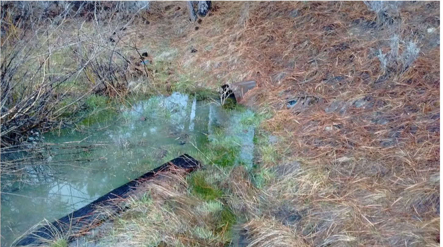
Previous photo and this one show the culvert on the north side of the balloon near the 2/3 switch. East culvert here is in the early stage of being undermined by creek.
