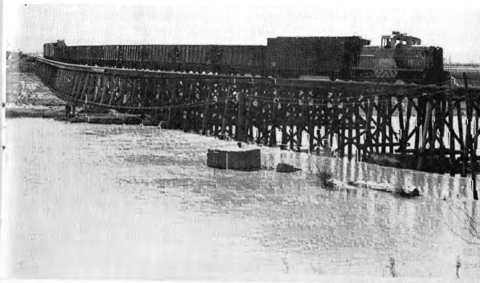
First train to cross the rebuilt Arcade trestle.
