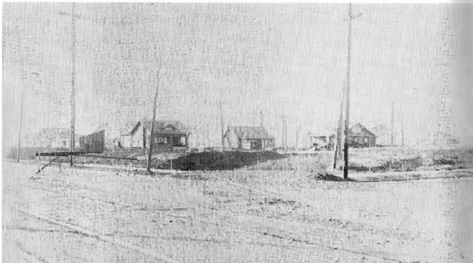
Looking northwest from the corner of 40th Street and Opal in 1912, a view of what is now the SN yards at 40th Street and Shafter Avenue, Oakland. Some of the houses still stand. —Vernon J. Sappers collection
