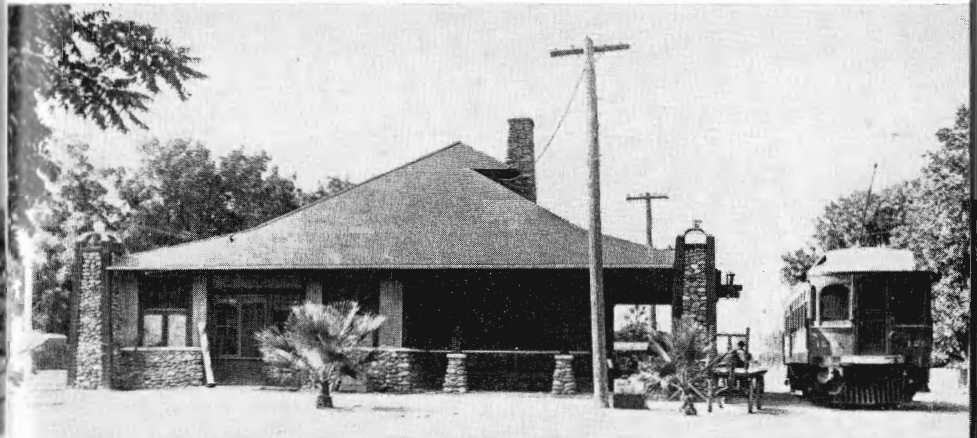
If there was no business at Pleasant Grove, trains would many times coast under a one-half mile of overhead wire between stretches of third rail, eliminating the raising or lowering of trolleys.
