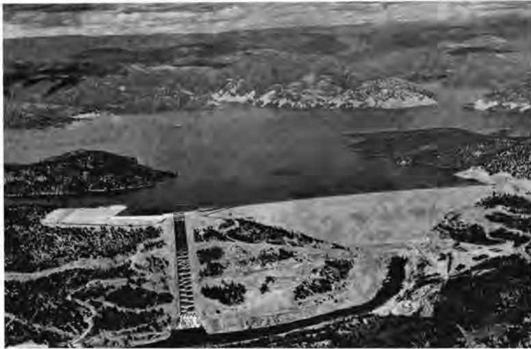
Oroville Dam on the Feather River about 5 miles northeast of Oroville is 770 feet high and will impound 3 1/2 million acre-feet of water. Carved from solid rock within its left abutment is largest underground powerplant in the nation. Roadway across top leads to spillway, parking area for 2,000 boats and trailers, and boat ramps. Lake Oroville has 167 miles shoreline.
