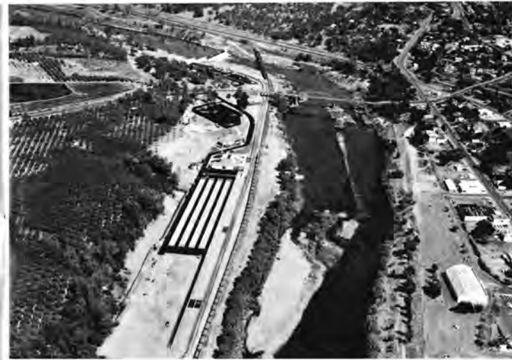
Aerial view of $3 million California Department of Fish and Game Feather River Hatchery, world's largest for salmon and steelhead. Photo shows fish barrier dam in background and portions of the City of Oroville on each side of the Feather River. WP's main line runs diagonally across top of picture beyond river.
