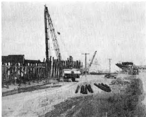
Construction work on the new trestle.
