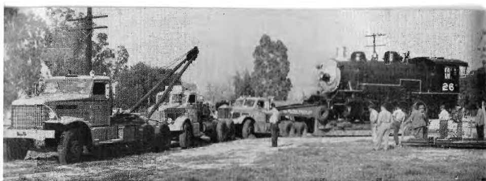
No. 26 made the last part of her trip from Glendale to "Travel Town" transported by the Belyea Truck Company as a free public service. She traveled Santa Fe Stockton to Los Angeles, SP from there to Glendale.
