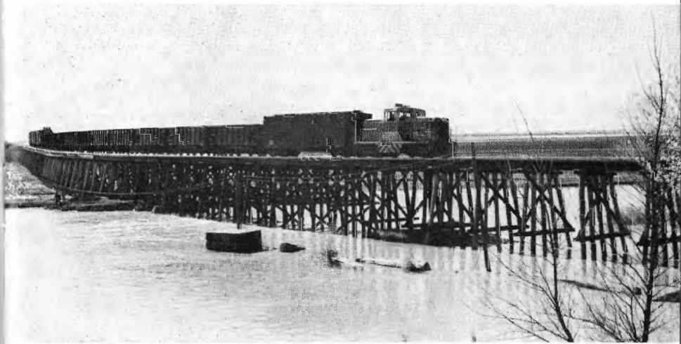
First Sacramento Northern train crosses the new trestle on April 6, 1954.
