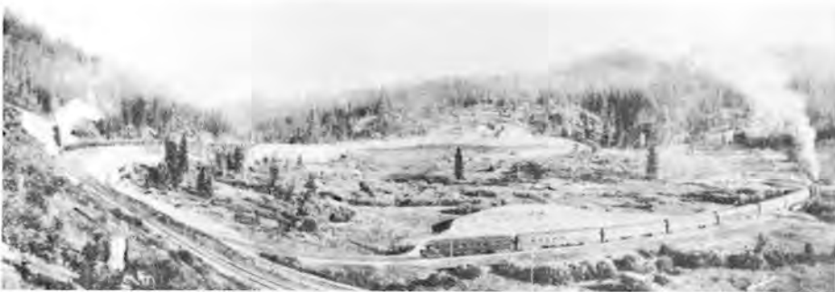
Williams Loop in the early days, showing the "cut-off" by which descending westbound trains avoided going around the circle.
