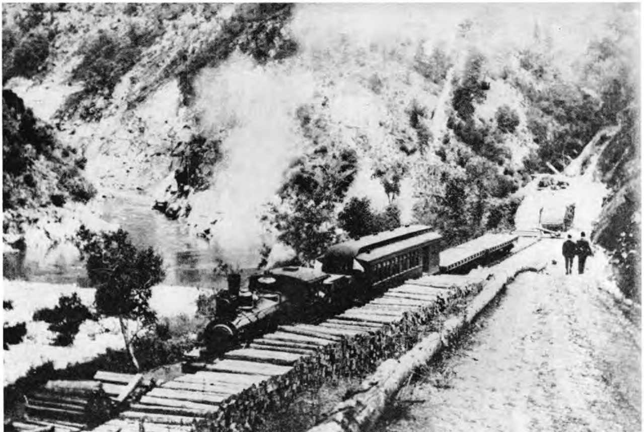
End of track at Berry Creek on May 17, 1908.
