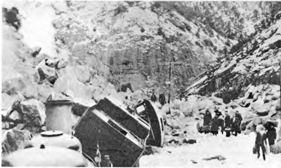
The Canyon was not tamed with the driving of the Last Spike. Until slopes had been scaled back and insecure boulders minimized, incidents like that above at M.P. 246 made the locomotive engineer's job similar to the airline pilot's of today.
