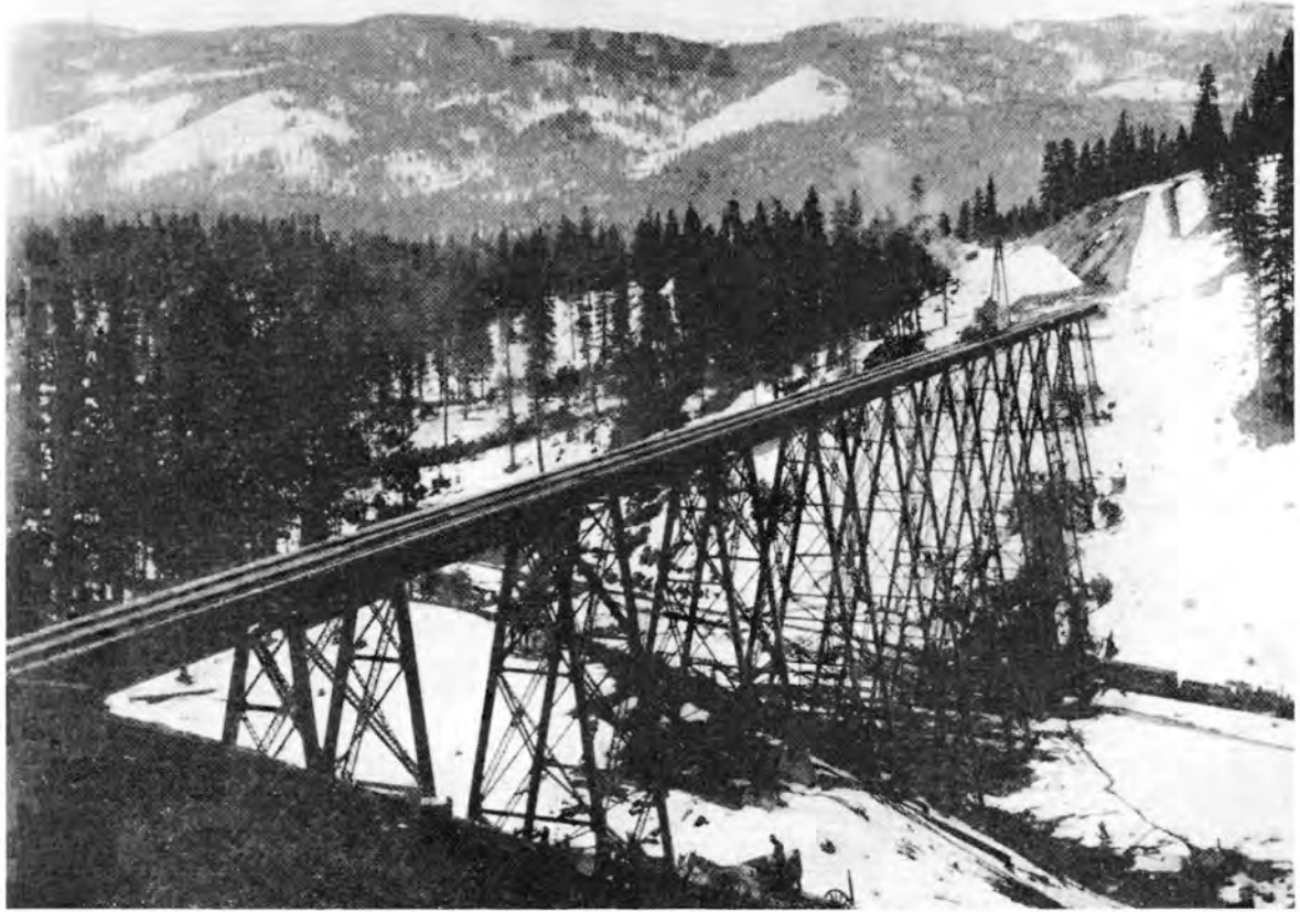
Construction of Willow Creek viaduct, 1,005 feet long and 172 feet high. Below is a train on the Sierra Valleys narrow gauge railroad.
