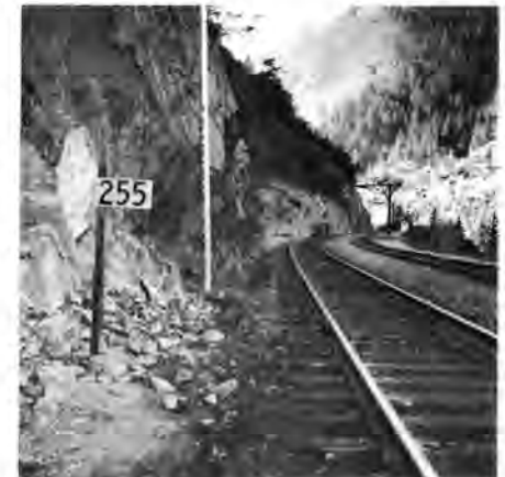
MILEPOST 255: Looking west from Camp Rodgers. Note the slide fence at the left and a portion of the 6713 foot siding at the right.
