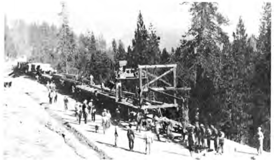
Below, "Improved Harris Track-Layer" putting down rail near Hartwell (now Quincy Junction).
