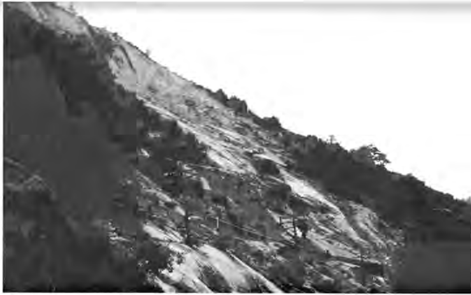
Site of slide at MP 250 after service restored. Photo by J. T. Smith.
