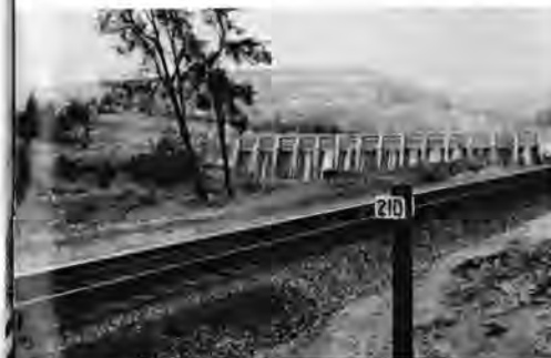
Milepost 210: After passing Thermalito diversion dam behind sign, main line first crosses Feather River over Feather River Bridge.
