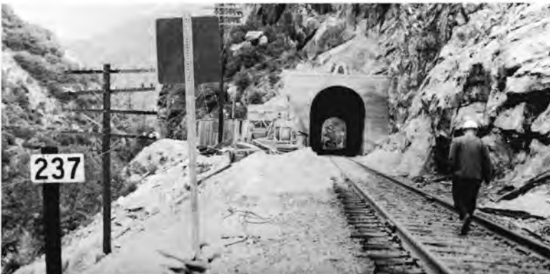
While Dave waited at Jarbo passing track for track time Maury took off on foot for closeup inspection of right of way. West end of Tunnel 10 just ahead.
