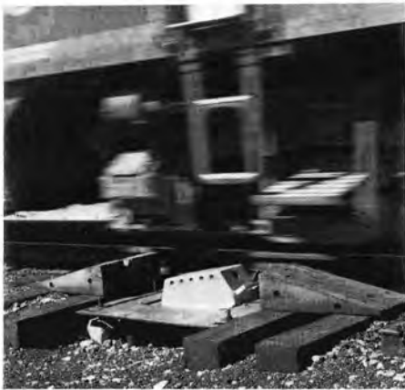
Heat from a hot box on the above passing freight car journal would be recorded by detector in foreground, received in Sacramento by carrier equipment shown at right, and recorded on graph being checked by Dispatcher Evan Neilson. Top picture taken by Special Agent-Claim Agent R. F. Stenovich; pictures below and at right taken by Signal Engineer Bruce McNeill, Jr.
