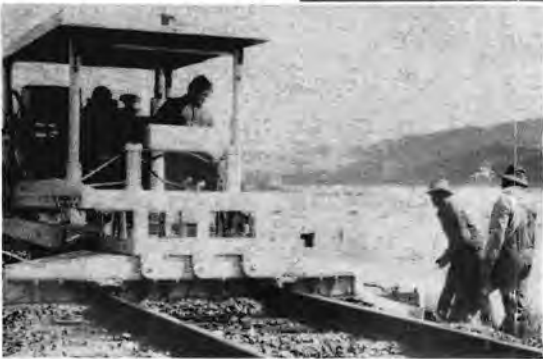
SCARIFIER- TIE INSERTER
