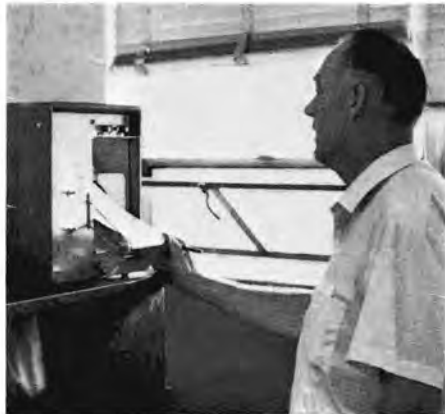
Heat from a hot box on the above passing freight car journal would be recorded by detector in foreground, received in Sacramento by carrier equipment shown at right, and recorded on graph being checked by Dispatcher Evan Neilson. Top picture taken by Special Agent-Claim Agent R. F. Stenovich; pictures below and at right taken by Signal Engineer Bruce McNeill, Jr.
