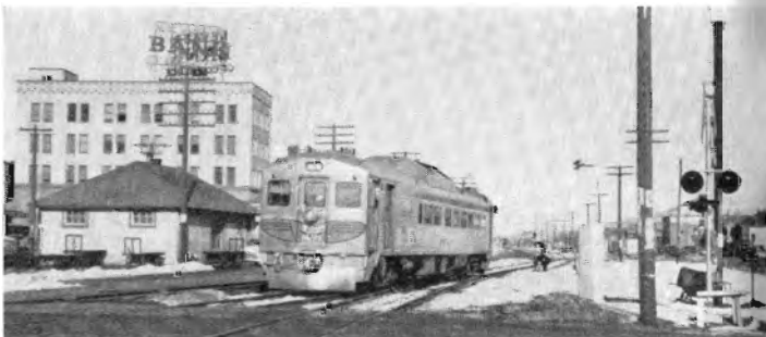
Passengers enjoy controlled heating, although snow is on the ground at Elko.
