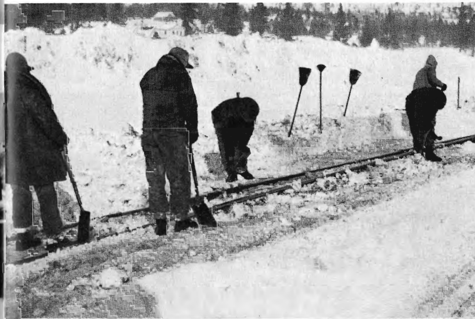
Constant shoveling by section forces kept the switches open for train operation in the yard. Rising winds blew drifts of powder snow over the tracks as fast as they were cleared.
