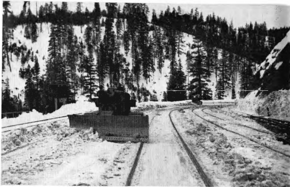
After the rotary plowed paths through the deep snow at Keddie, and flangers further cleared the tracks, bulldozers pushed aside remaining piles of snow on January 23.
