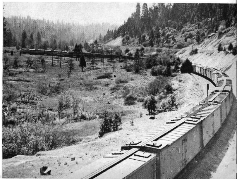
To maintain the easy 1 per cent grade, Western Pacific's main line makes a complete loop in the upper end of the Feather River Canyon. This long freight, headed by diesel power, is shown headed east around Williams Loop.
