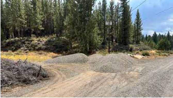
90 Yards of Rock for Work on the Balloon Track - Photo by Roger Stabler
