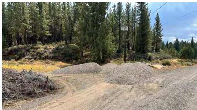
90 yards of new ballast for balloon track. - Photo by Roger Stabler
