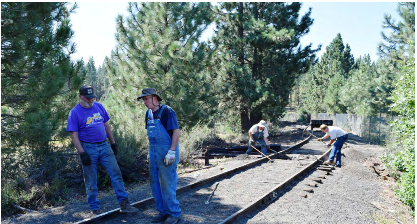
Bil Jackson and Roger Stabler discuss tamping needs on 9 August 2017 as Ethan Doty and Jason Peterich prepare the next tie insert location. Roger has repaired the tamper and has 6 of the 8 tamper motors working and two motors to install at a later date.
