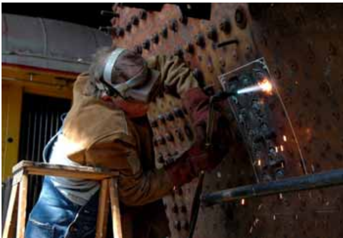
Jim Prettyleaf, GGRM welder, removes a wasted section of the 165's wrapper sheet.
