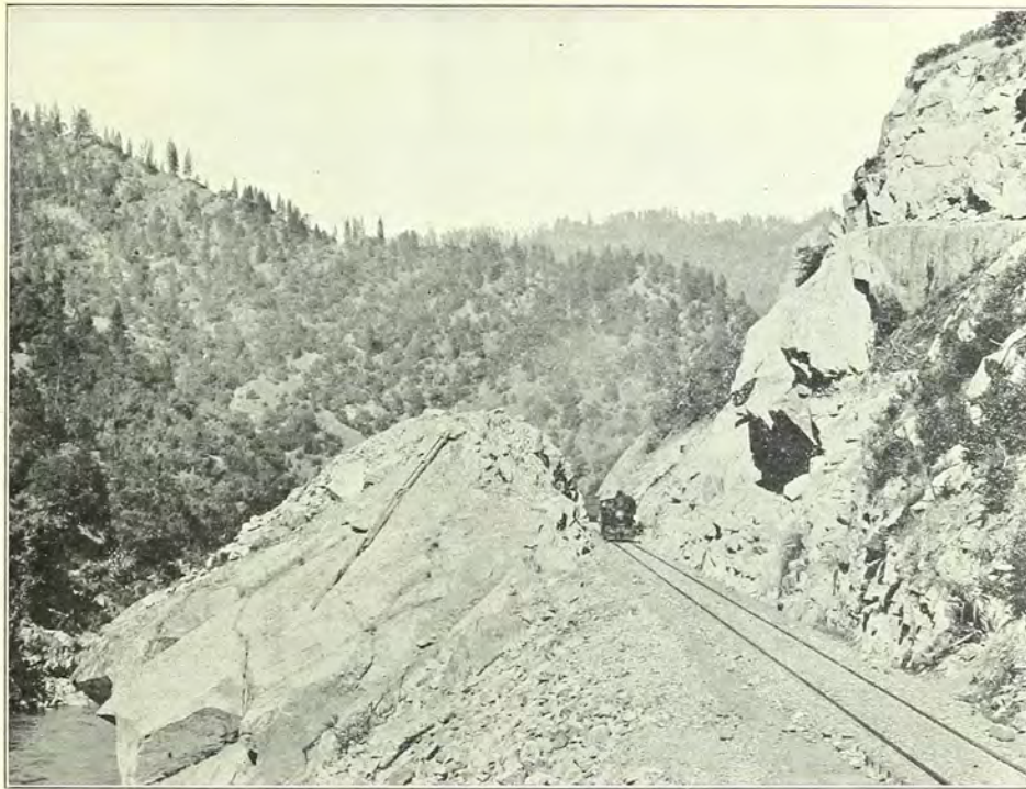
A BIT OF HEAVY CONSTRUCTION, SHOWING ALIGNMENT
