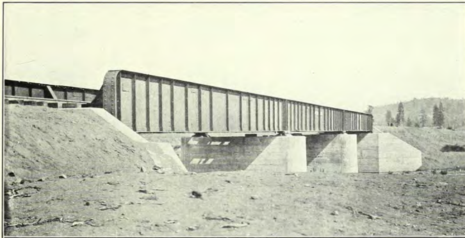
TYPE OF PLATE GIRDER BRIDGE
