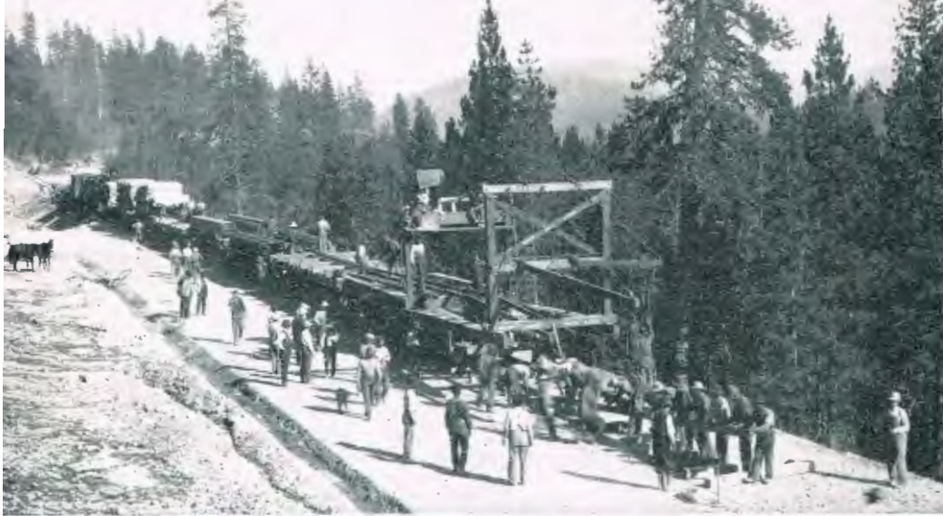
The most modern techniques were used in building the Western Pacific. Here the "Improved Harris Track-Layer" is seen putting down rail near Hartwell (now Quincy Junction).
