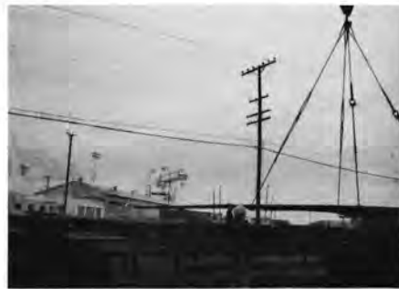
Huge cranes were used to off-load plates, in preparation for placing them aboard railroad cars.
