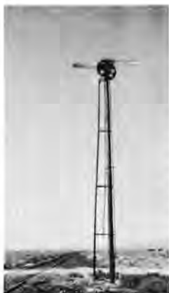
Old Nevada Northern R.R. train order semaphore at Shafter, Nevada as she looked in 1973. This signal was installed in 1908 and was operated by WP employes at the WP-NN crossing at Shafter, Nevada.
