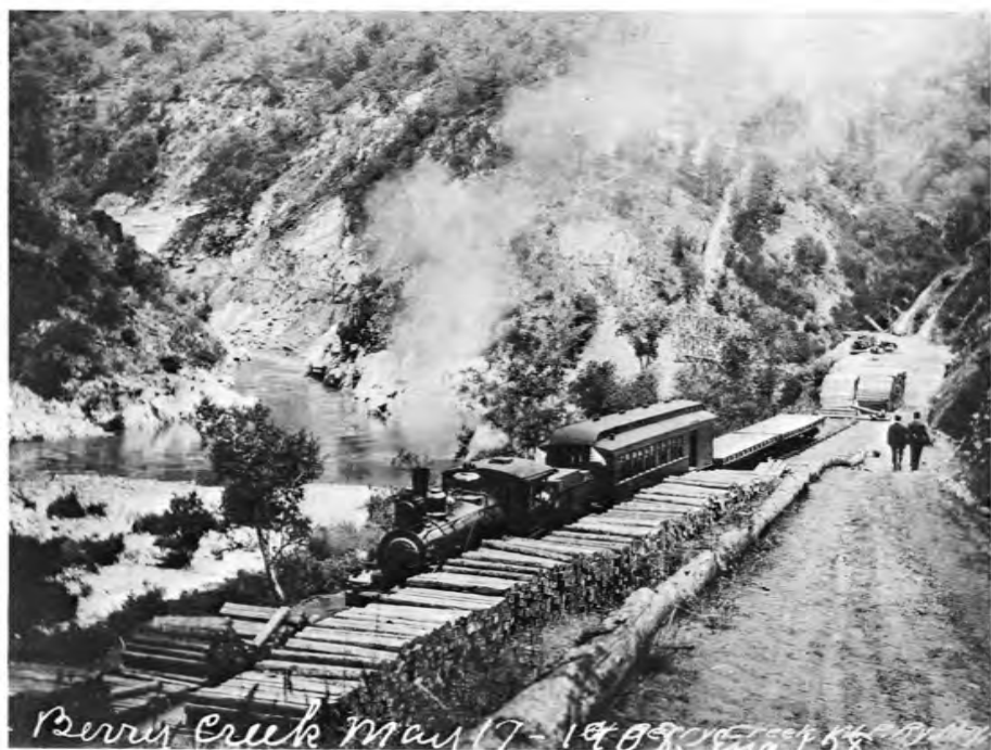
The view at the end of track at Berry Creek, Ca., on May 17, 1908, showing a stockpile of ties to be used in construction. Berry Creek is milepost 225, 20 miles east of Oroville.
