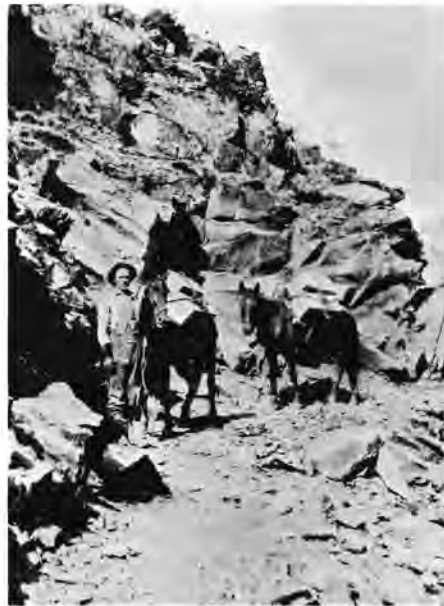
In advance of the track gangs, blasting powder was brought into the more remote arcs of the Feather River Canyon by pack horses.
