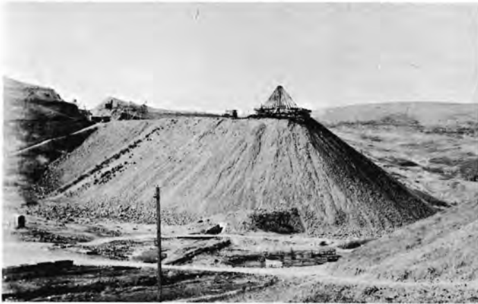
The "Merry-Go-Round" was used in constructing large fills at milepost 59.
