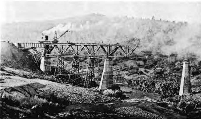
This photo taken in November of 1907 shows the construction of bridge # 212.36, the middle fork crossing, 7 1/2 miles east of Oroville.
