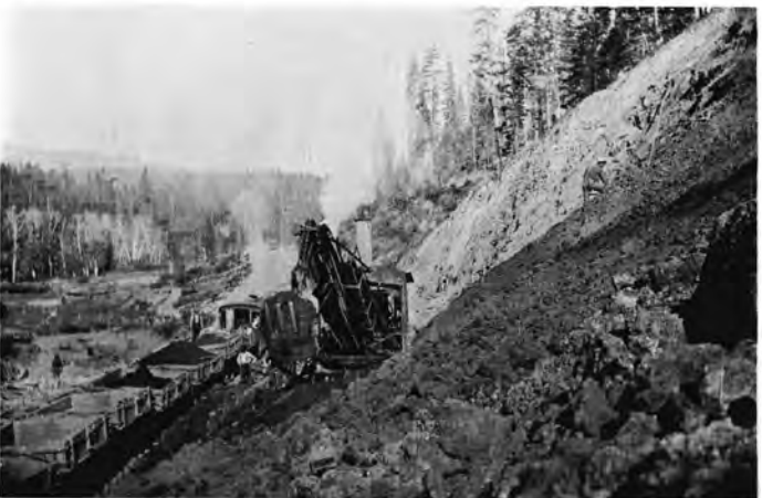
A steam shovel aids in the track construction on the Sierra Division of the WP in 1907. Western Pacific, unlike earlier transcontinentals, was largely machine constructed, though the equipment used seems quaint by today's standards.
