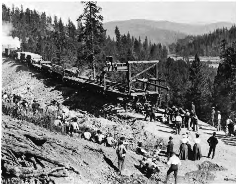
The "Improved Harris Track Layer" drew many on-lookers as it put down rail near Hartwell (now Quincy Junction, Ca.) in the fall of 1909.
