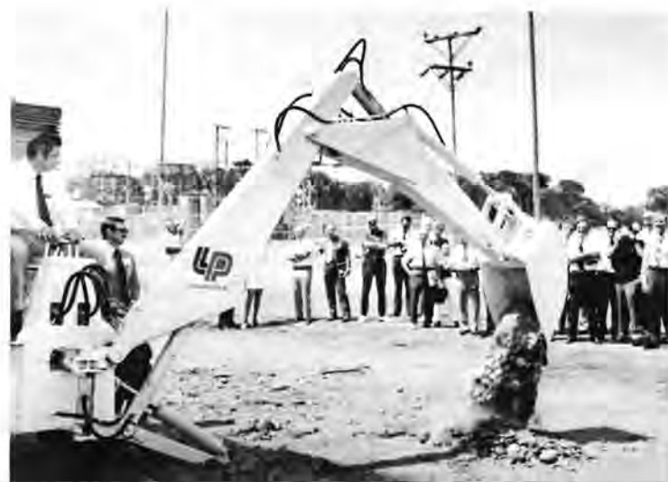
Louisiana-Pacific President Harry A. Merlo breaks ground with backhoe as Plant Manager Sherman Kirchmeier and guests look on.
