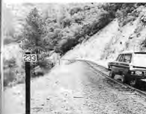
Milepost 233: First milepost sign one mile east after leaving new main line.
