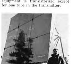
Lineman Ed Nay (above) cleared the brush and trees obstructing line-of-sight path of reflector on Beckwourth Mountain. Reflection of tree is shown on reflector's surface. It must remain flat within 1/2-inch overall, even during 100 mile per hour winds.
