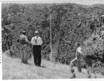
Looking west with Tunnel 5 in the center of the picture from Highway 40-A, Milepost 230.6. Despite rugged country, new line will be about four miles shorter than present line. In addition to tunnels and bridges, many cuts and fills will be required to maintain the railroad's present grade.
