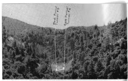
Driving of Tunnels 4 and 5 is expected to begin this month. Passengers will get only a glimpse of Dark Canyon at Milepost 230.4 as their train emerges from the 4,412-foot Tunnel 4 before entering the 8,830-foot Tunnel 5. Between these portal entrances the line will cross on a 65-foot concrete arch bridge.
