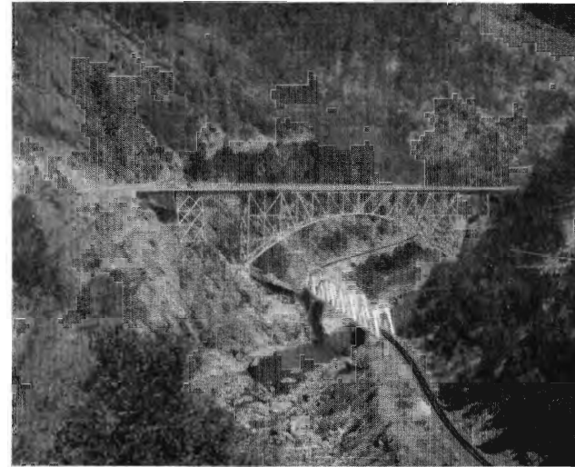
Looking down from high above, railroad and highway bridge overhead form huge "X." This picture was taken by Jim Lindsey, member of Paint Gang No. 1.
