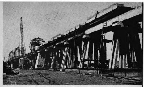
New bridge is higher and more strongly constructed to withstand future flood damage. Note pre-cast concrete girders atop flatcars ready for placement by gantry crane.
