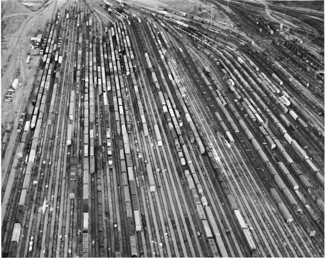
Union Pacific's North Platte, Neb. yard, the largest classification yard in the world, has a capacity to dispatch 50,000 tons of freight each day.
