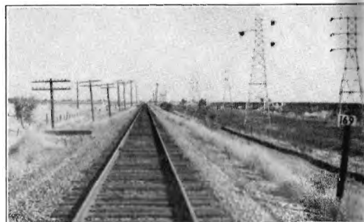
*Milepost No. 169: Looking east about midway between Trowbridge and East Arbogo.
