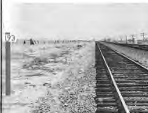
Milepost 193: In vicinity of Craig. On right is 125-car capacity passing track.
