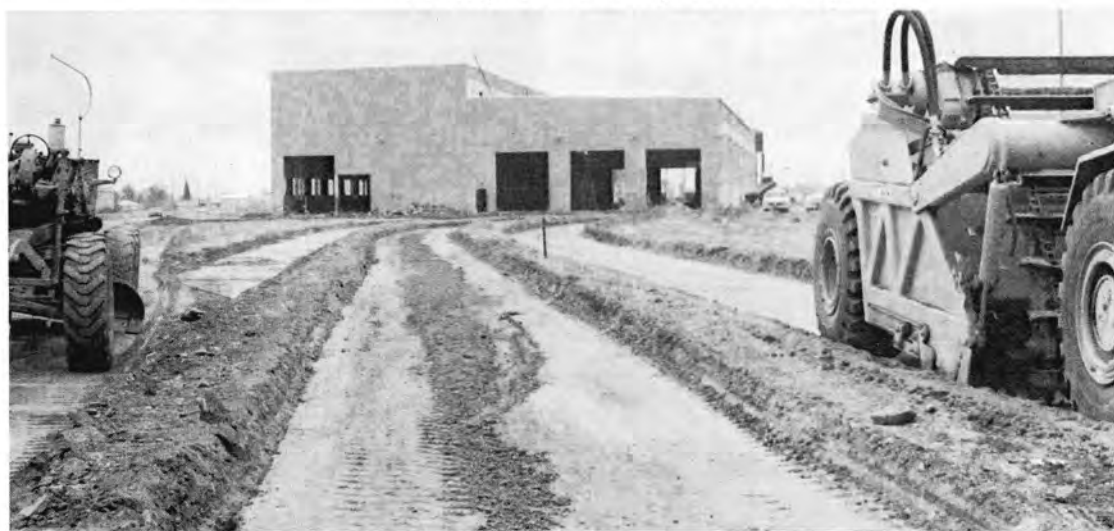
Stockton locomotive maintenance facility nears completion—Page 3
