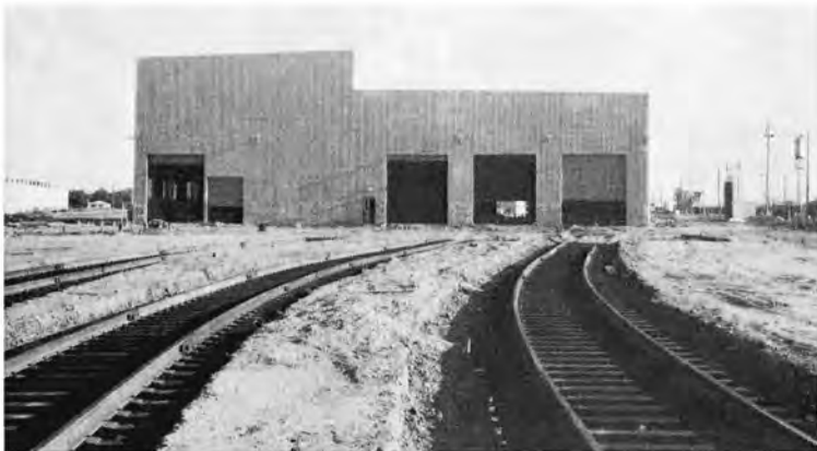
Three tracks will run through building's service bay at right. A single track will enter but not pass through repair bay on left. Photo by John Sterner, special agent and claim agent.
