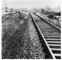
Looking east along replaced main line track. BARTD track will be at grade level at left in area occupied by temporary shoofly track.
