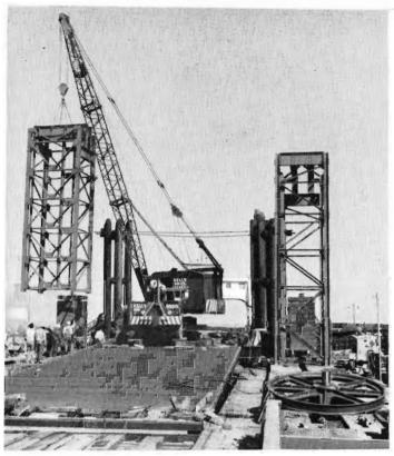
Left: Kelly Bros. crane with shortened boom drops gallows frame over counter weights. Bull wheel, right foreground, is one of two used to support main cable for lifting apron.
