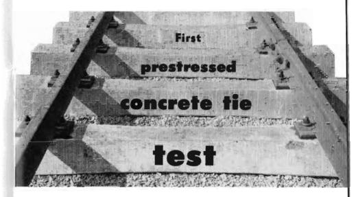
Western Pacific, simultaneously with two railroads in Florida, installed during March a number of prestressed concrete track ties for test purposes. This represents the first use of this type tie in this country, although standard reinforced concrete ties have been used by American railroads as far back as 1893.
