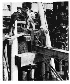
Right: Nordstrom, left, directs driving of prestressed concrete pile between wooden piles left in place. B&B Carpenter S. J. Davis watches progress from below, assisted by two unidentified workmen, above center.
