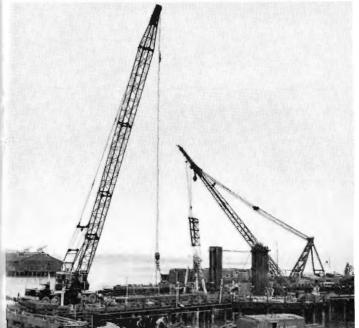
Truck-mounted crane at left, owned by Kelly Bros., San Jose, is one of the largest of its kind on Pacific Coast. Long boom was necessary to permit crane to operate from dock while apron was being dismantled, Gerwick's barge crane lowers pile driver leads into position.
