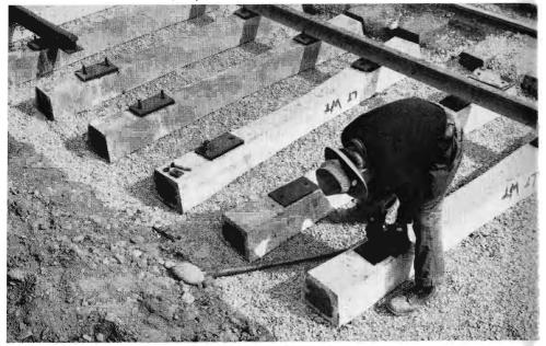
Completed installation except for ballasting; first four rows of ties in foreground are wooden cross ties. The 45 prestressed concrete ties used for the test installation were placed just in front of the timber trestle, shown in the distance just in front of the new apron.
