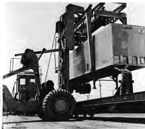
WP's huge side porter eases a trailer onto a flatcar at Oakland yard for WP's new TOF train leaving about midnight. Carrying only trailers/containers the train makes 23½-hour run to Salt Lake City five days a week.
