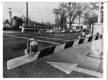
An electronic solid state analog controller computed the speed of this California Zephyr as it approached the crossing, placing gates in operation to protect vehicular traffic.
