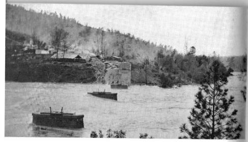
Magnitude of the Feather River flood of March, 1907, is shown by the construction photos of Bridge No. 112.36, the Middle Fork crossing 7½ miles east of Oroville. The upper shows the bridge viers barely clearing the crest; the lower was taken the following November, with the river at its normal flow.
