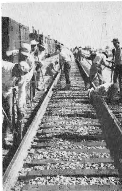
A 388-mile haul of one ton of freight would be required to buy each spike, tie plate and treated fir tie being installed by this gang of track workers.
