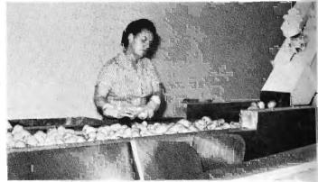
Razor-sharp knives encircle object shown on shelf which is one of several types placed inside potato slicer just above which, operating at extreme high speed, slices potatoes to a uniform and exacting thinness before frying.
