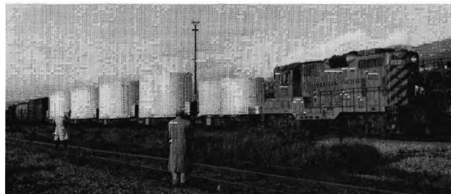
Two photographers record first shipment of UTC booster rockets in WP train as they leave Milpitas on 2,900-mile trip to Cape Kennedy.
